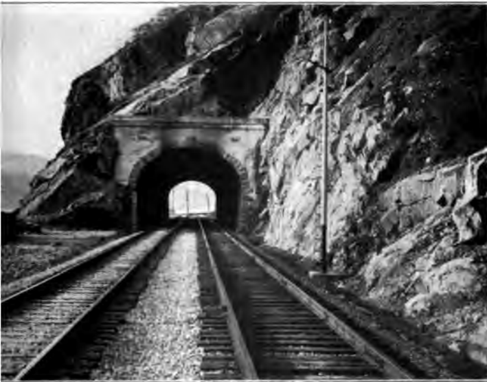
REVISION ON THE NEW YORK CENTRAL — TUNNELLING THROUGH THE BASES OF THESE JUTTING PEAKS ALONG THE HUDSON RIVER DOES AWAY WITH SHARP AND DANGEROUS CURVES
